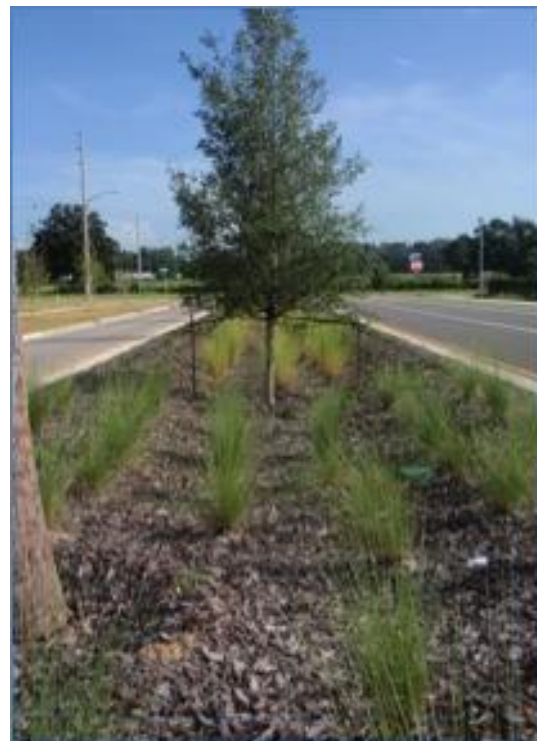
Figure 5.6.2. Schematic and Photo of Rain Garden
