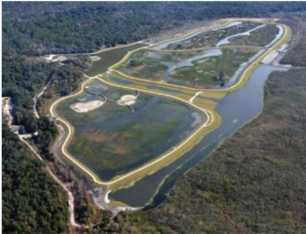
From: Paynes Prairie Sheetflow Restoration Project presentation, Alice Rankeillor, P.E. GRU, 2015
