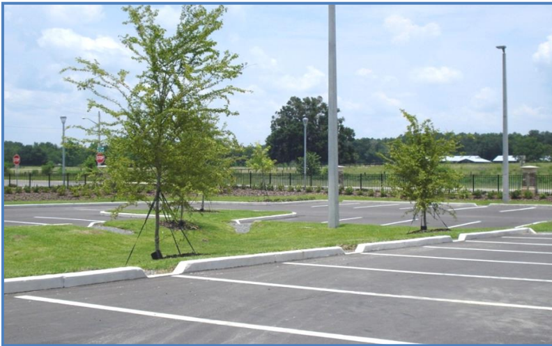
Curb cuts at Campus USA Headquarters in Alachua County allow runoff to flow into depressed island retention areas
